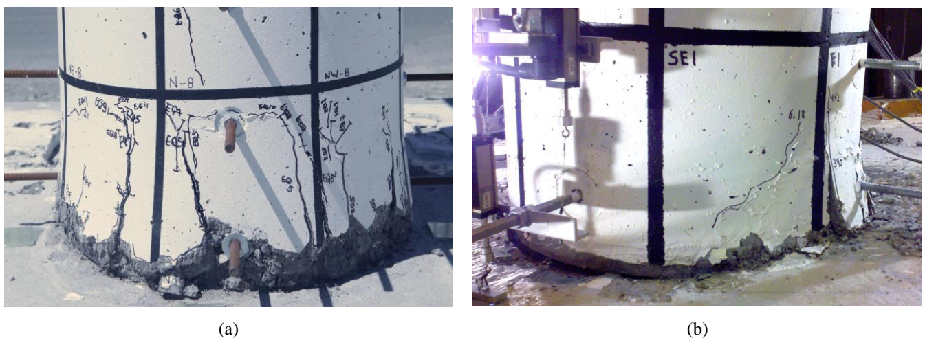
Fig. 3 – Compression damage in rocking HPFRCC bridge columns: (a) After 11 tested ground motions (Trono et al. [12]); (b) During loading cycle with a peak drift of 11.3% (Nguyen et al [14]).
